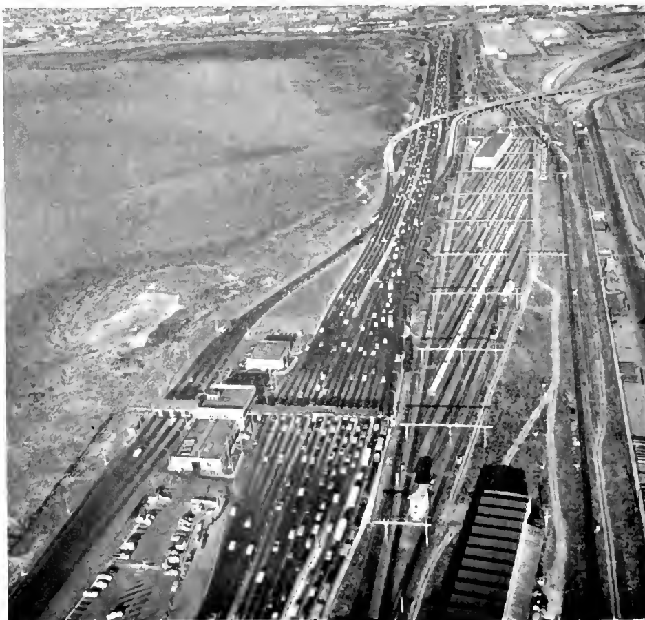
Close-up of Toll Plaza looking easterly. Note the idle railway rolling stock in storage yard adjacent to toll gates. Vehicular traffic passed through the toll gates in record numbers. The toll collection staff did a remarkable job under difficult circumstances as evidenced by the fact that collectors handled daily, during peak hours, as many as 12 cars per minute, or one car every five seconds.
